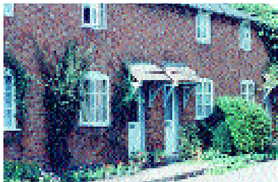
Lean-to canopies on brackets, Welford-on-Avon, Avon Valley area. The roof material in this case is inappropriate
