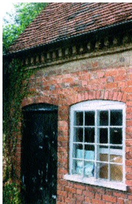
Variation of dentilated brick eaves with alternating projecting headers on edge, also showing a rise-and-fall gutter fixing, Great Alne, Arden area
