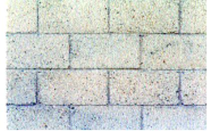
Concrete block wall
