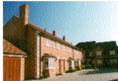
Two different house types used to make the best of a long narrow plot in a new development off High Street, Henley.
