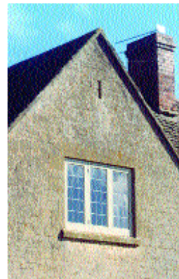
Plain eaves, trim verge and mortared ridge on a Cotswold Limestone house, Great Wolford, Cotswold Fringe Area
