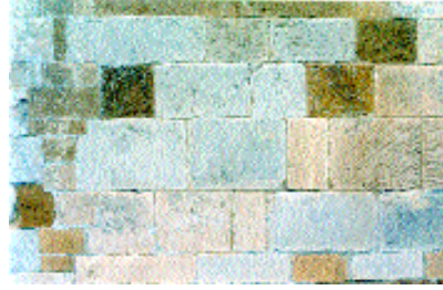
Ashlar wall of Cotswold limestone and Hornton marlstone
