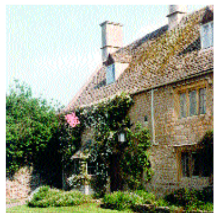
House in Cherington. Local stone has been used for the walls, roof and boundary wall.
