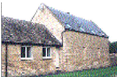
Sensitive conversion in Long Compton with simple, restrained flush closing casement windows and rooflights set flush with the roof.
