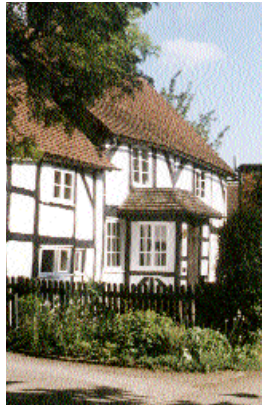
A boundary with planting and pale fence, Tanworth-in-Arden, Arden area
